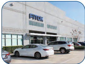
FITOK, Inc. Manufacturing & Global Sales Center - Texas, USA
